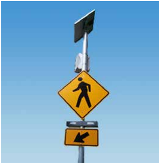
Crossing enhancements, such as crossing beacons, reduce vehicle speeds approaching the crossing point, which help to improve safety and mobility.
