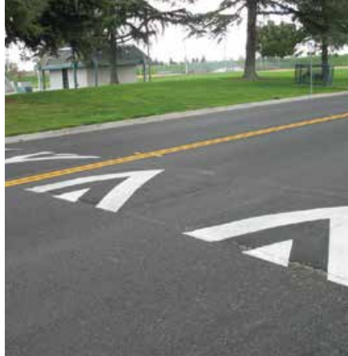
Speed humps can be effective at reducing speeds and diverting traffic to adjacent streets.
