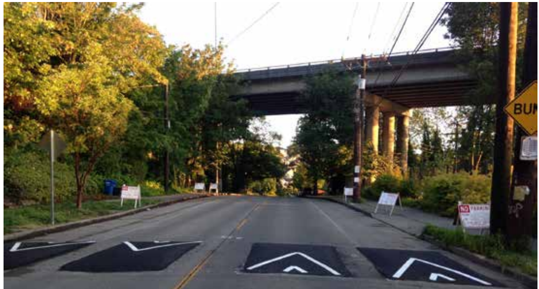
Newly installed speed cushions on Boyer Avenue East.
